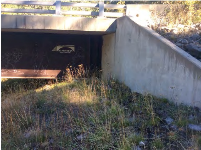
Right Bank Abutment when facing downstream
