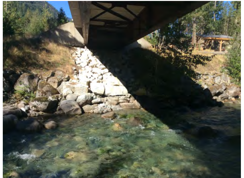
Right Bank Abutment when facing downstream
