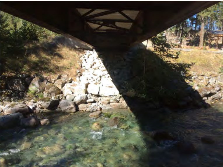
Right Bank Abutment when facing downstream
