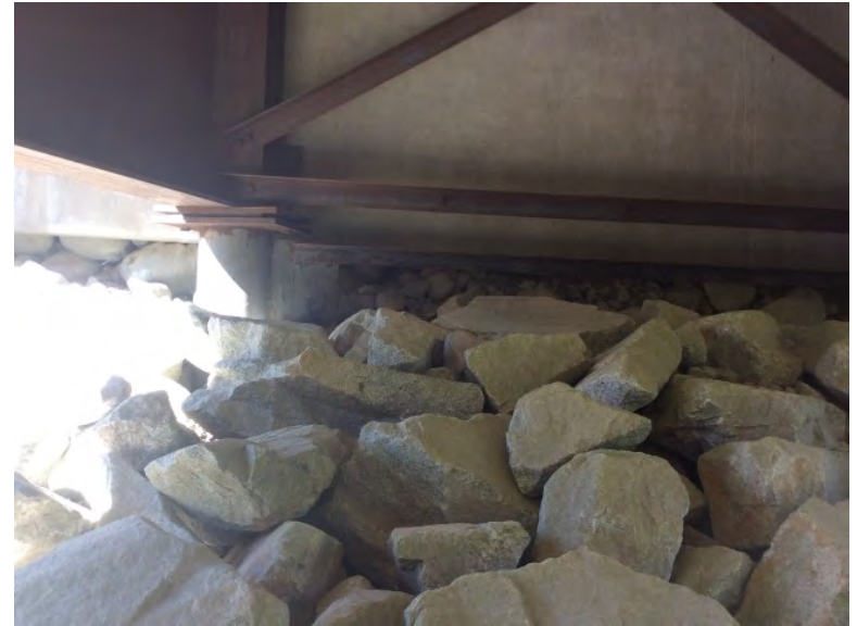
Right Bank Abutment when facing downstream
