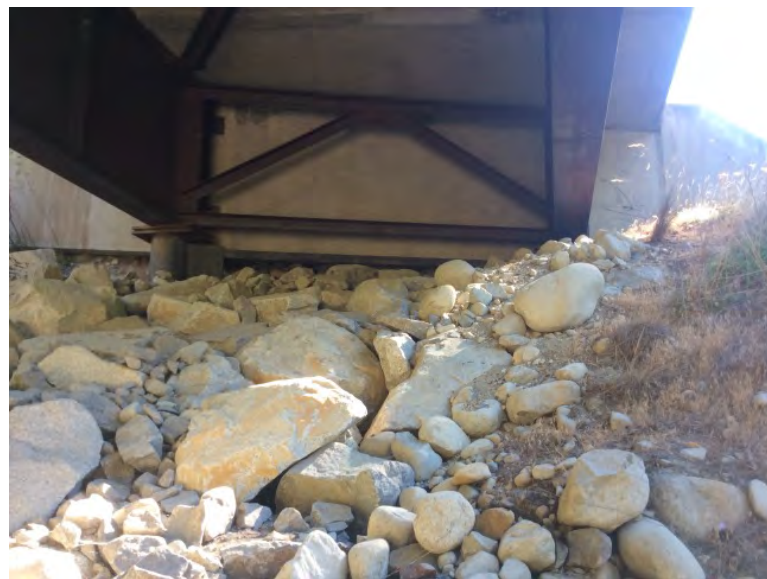
Right Bank Abutment when facing downstream
