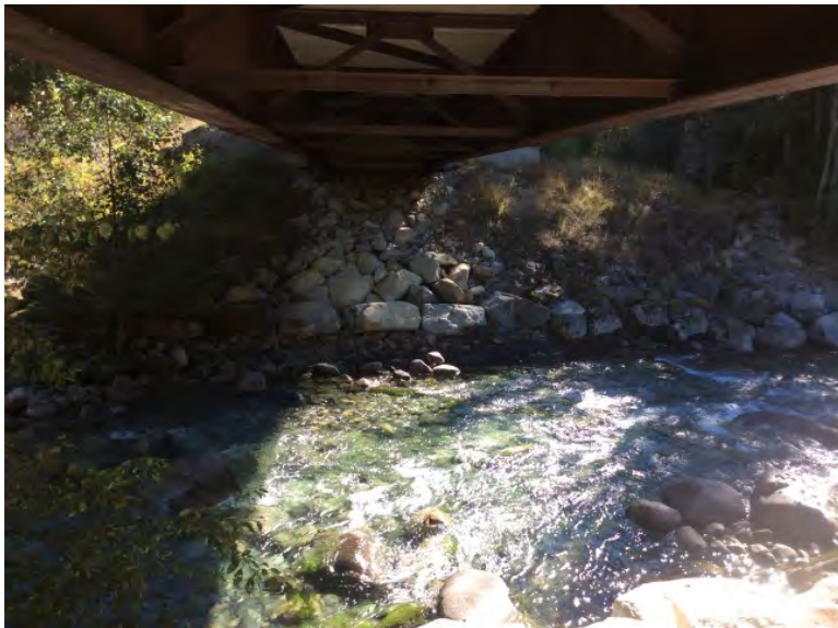
Left Bank Abutment when facing downstream
